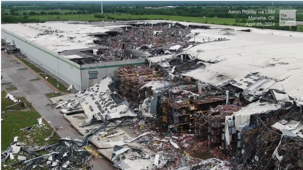
A Dollar Tree warehouse in Oklahoma after a violent EF4 tornado in April 28, 2024.
